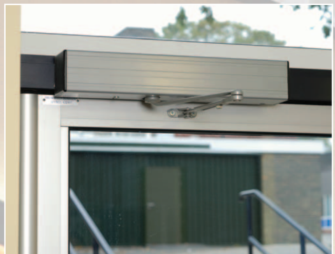
LCN Auto Equalizer for controlled disabled access Maiden Erlegh School, Reading
